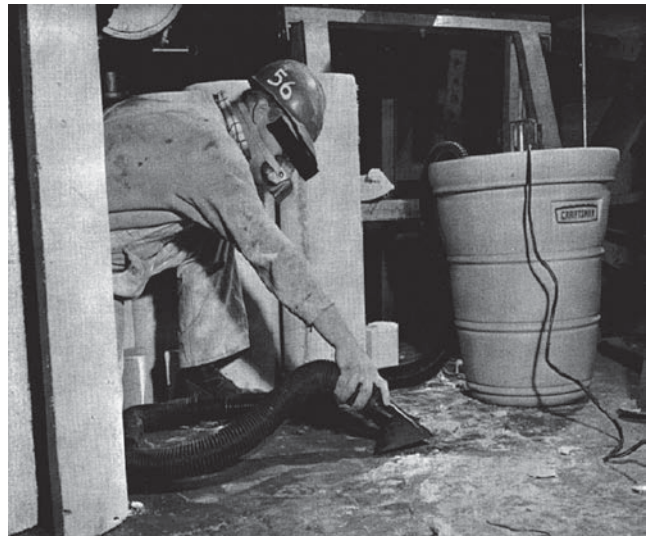
Figure 8. Worker cleaning work area with a vacuum, while wearing a respirator. Photo source: Carl Mangold. Previously published in Hollins et al., 2009.
